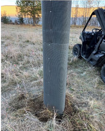
Images: Pole fire wrap (left) covered conductor (right)
