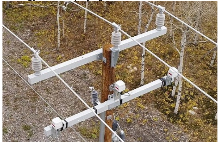
Image: lower arms of distribution pole show the early fault detection technology used.
