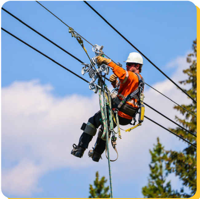
Spaced Aerial Cables help keep lines stable during high winds, while covered conductors provide a barrier between energized lines and nearby vegetation, fallen trees or small animals.
