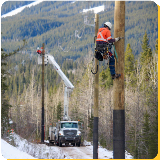
Fire wraps help protect power poles from fire damage.
