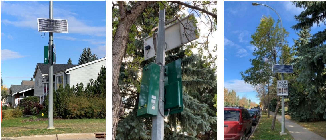
Figure 4: Solar speed signs on streetlight poles
