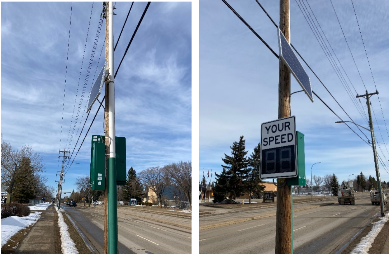
Figure 7 – (NOT ALLOWED) Speed signs restricting access and encroaching on communication zone
