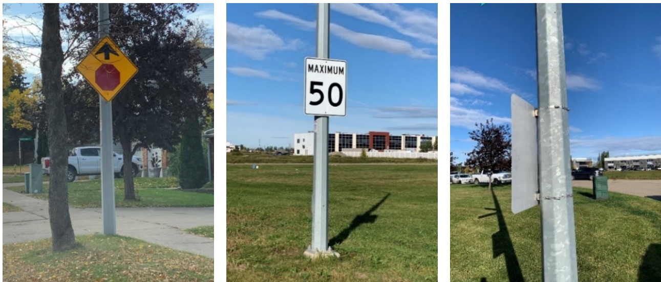
Figure 5: Traffic and speed signs on streetlight poles
